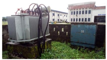
Fig. 4. 500kVA, 11/415V Transformer situated at College of Technology.
