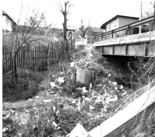
Fig. 6. Undimensioned and unkempt bridge over Helegiu creek, (Helegiu village).
