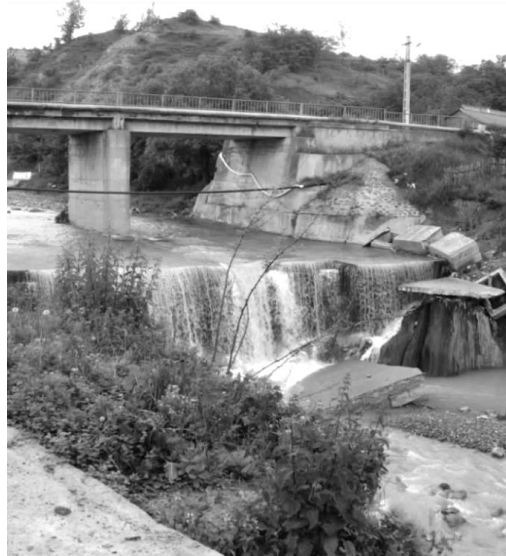
Fig. 4. Erosion accentuation, in depth, downstream of the concreted part of the bridge at Lucacesti (Tazlaul Sarat River).
