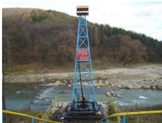
Fig. 5. Gas exploitation unit in Targu Ocna.
