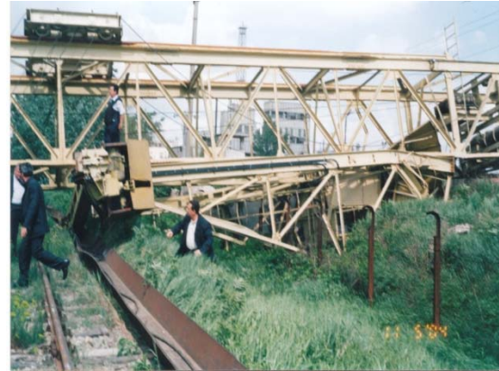
Fig. 2. The crash of the crane. Detail.
