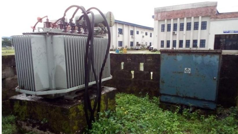
Fig. 4. 500kVA, 11/415V Transformer situated at College of Technology.
