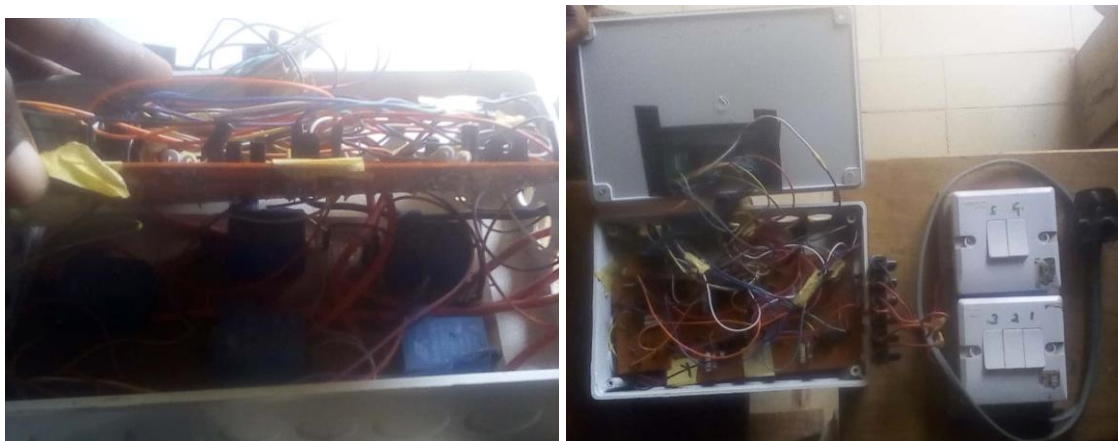
Fig. 16. Hardware implementation of the system.
