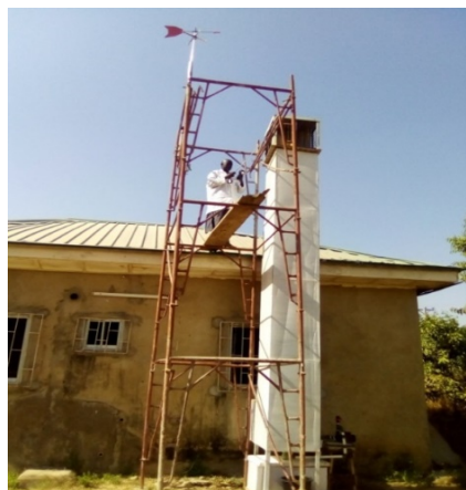
Fig. 5. HDEC integrated to office building.
