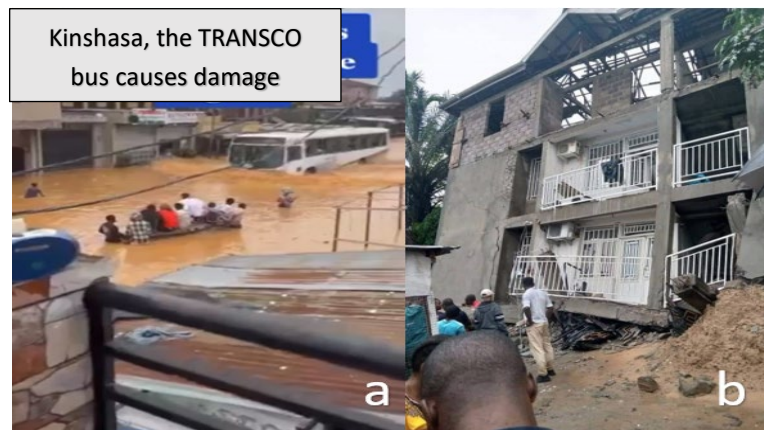
Fig. 2. Images from the affected zone: a) a bus is driving on a flooded road; b) collapse of a building following a torrential rain.
